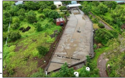
Fig. 2. Drone view of physical model
