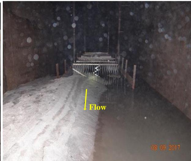
**Photograph 2.** High Sediment Deposition on RHS of wall in TRT
