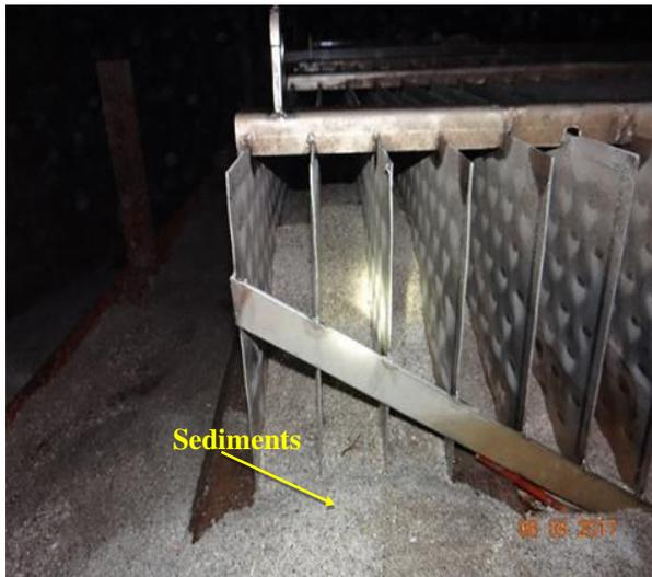
**Photograph 1.** Sediment Deposition in between econocoils of heat exchangers
